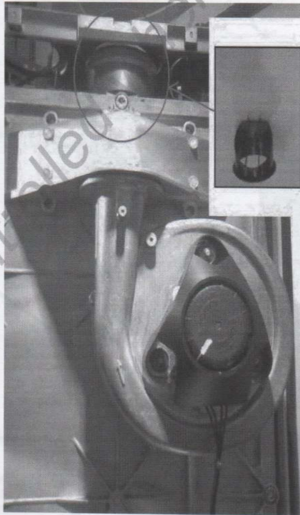
FIGURE 8 - TYPICAL POSITION FOR A NRV FITTED INTEGRAL WITHIN THE APPLIANCE
