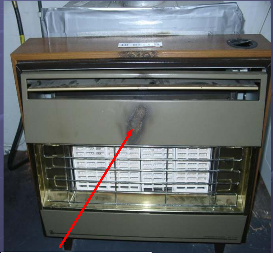
Signs of spillage
